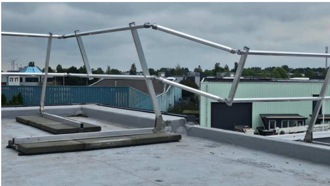
Finally double-check and tighten all bolts and connections before completion.
